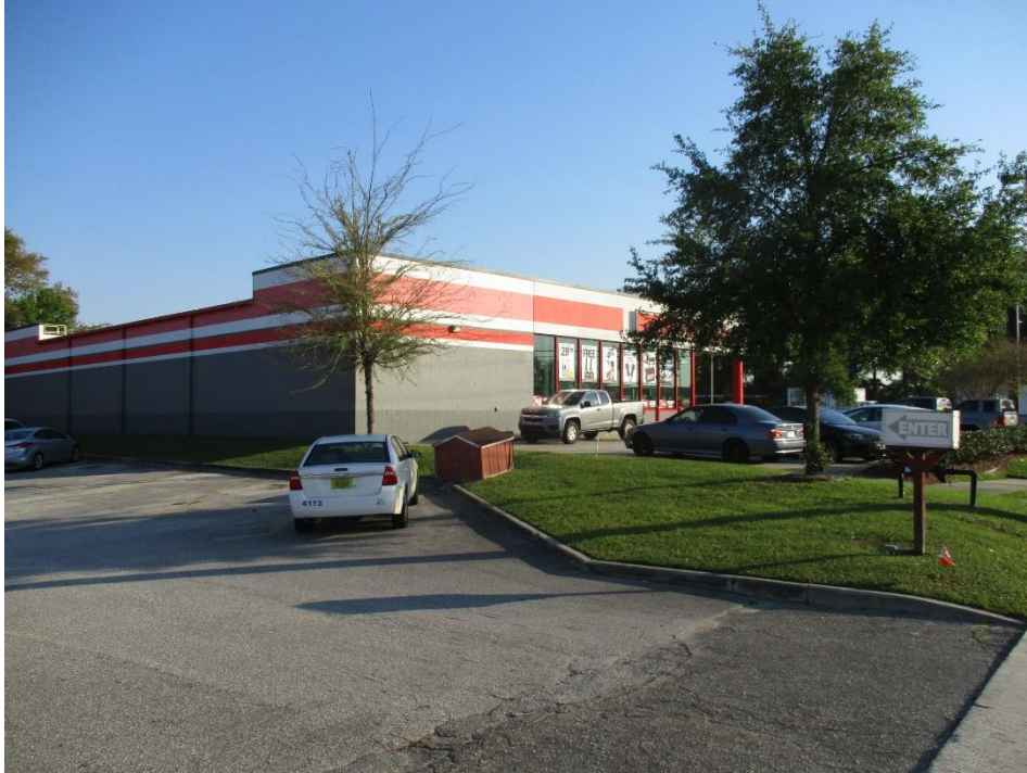
View of the neighboring property to the east of the subject property.
